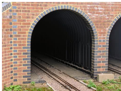
An example of a tunnel portal on a 7 1/4" gauge railway. Note the headroom and clearances.
